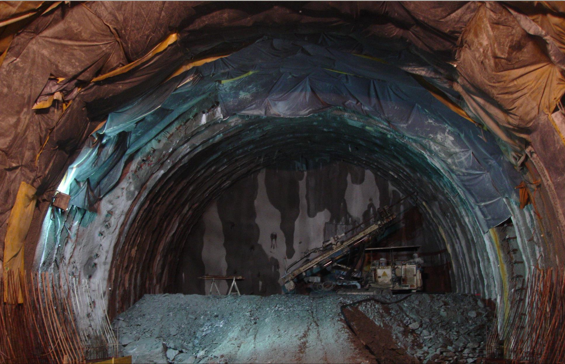
ROAD REHABILITATION WORKS BETWEEN ETROUBLES AND THE HIGHWAY JUNCTION FOR THE SAN BERNARDO TUNNEL | Italy
